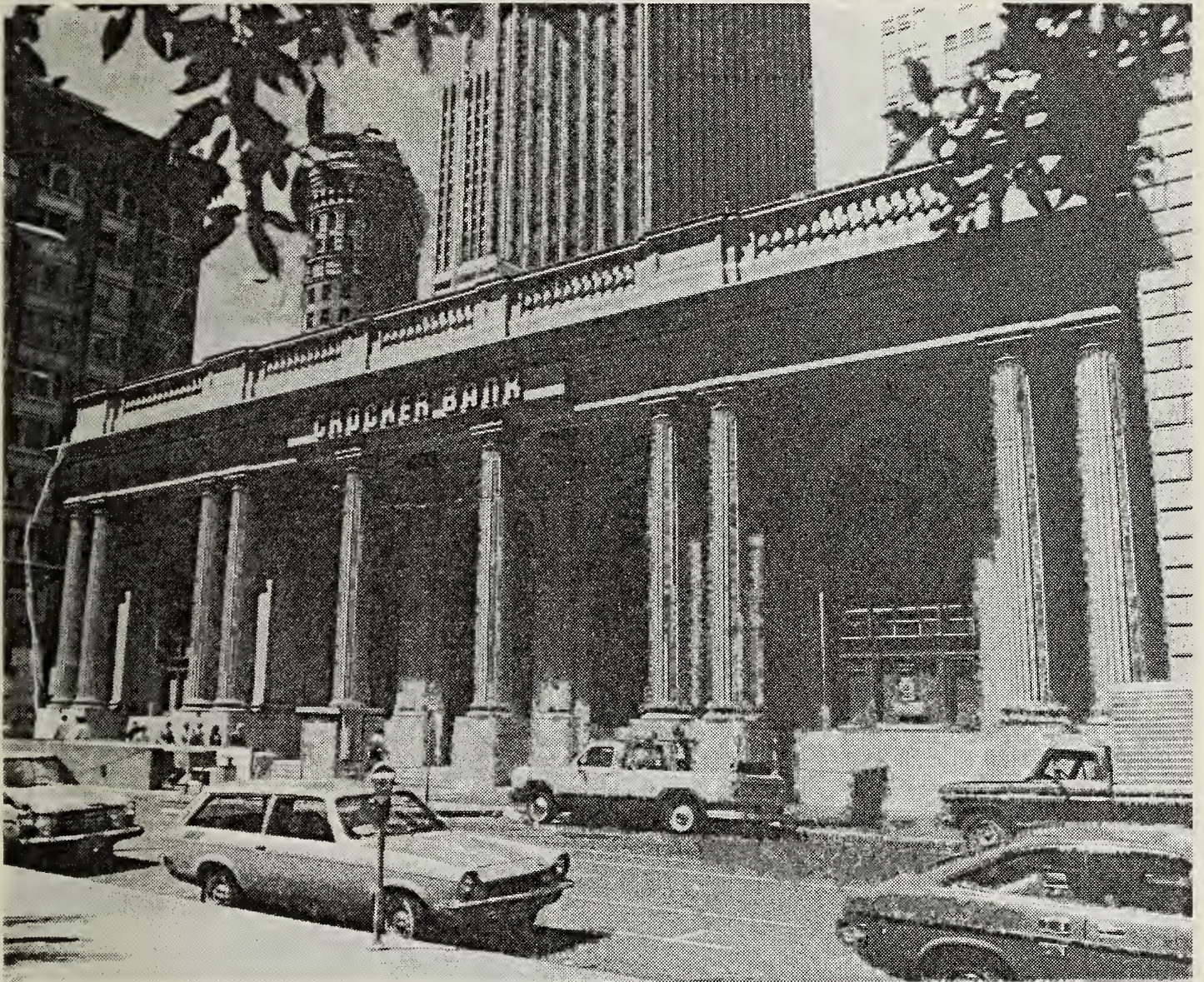
Note: Pissis' original entrance bay to the left, Kelham's addition of four bays on the right.
